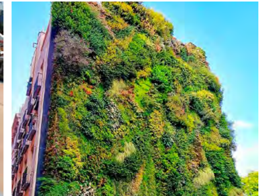
Frontage to Castle Park - Biodiverse Vertical Greening
