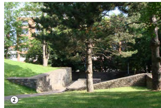
Fig. 94 Existing walls within Castle Park
